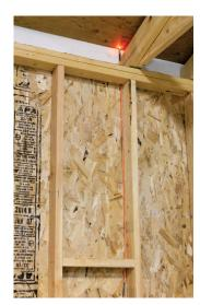
Using the light to guide you in the attic, snag the line with a Hook Tip mounted on another Fish Rod. Pull the line towards you.
