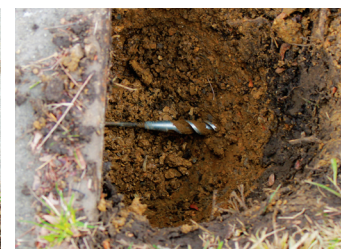
A small hole on either side of the sidewalk and a simple hand drill is all that is needed.
