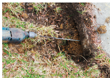
A small hole on either side of the sidewalk and a simple hand drill is all that is needed.
